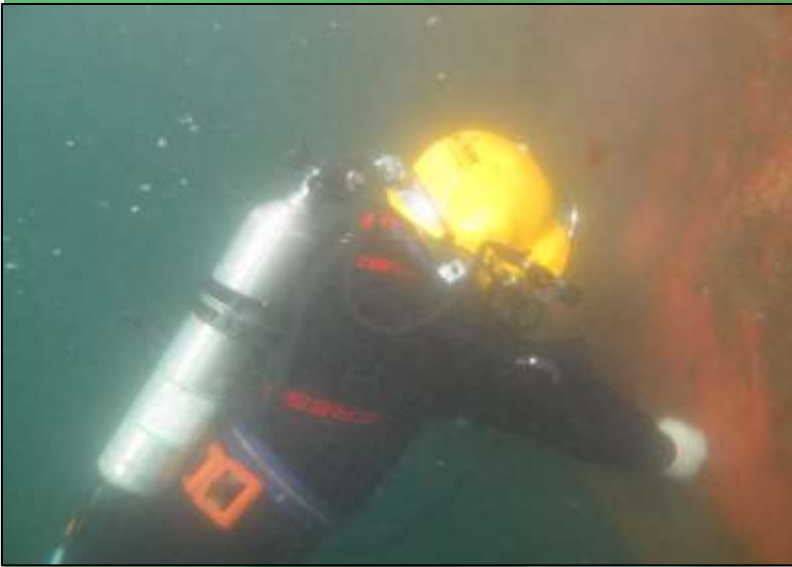
UNDERWATER CUTTING WORKS
